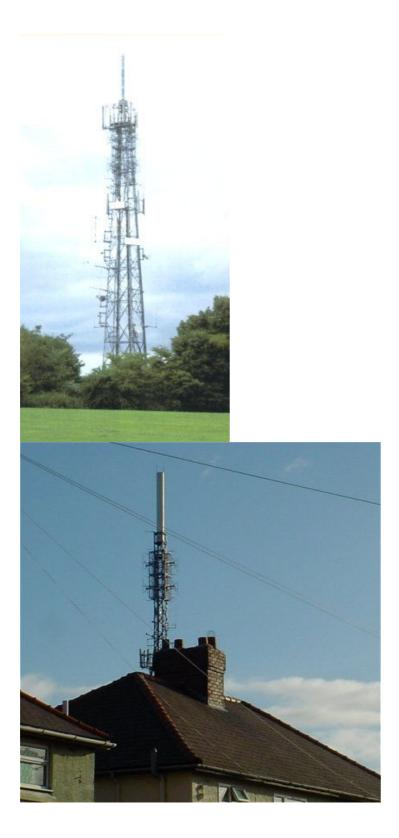
Each base station provides coverage over a limited area, or cell, in the area around the site. That's why in some countries mobile phones are called cell phones. To offer comprehensive network coverage, the cells must overlap each other like a patchwork quilt, so that users can move from one cell to another without breaking connection. As each cell can only handle a limited number of calls, the density of base stations has to be high in areas of heavy use.
